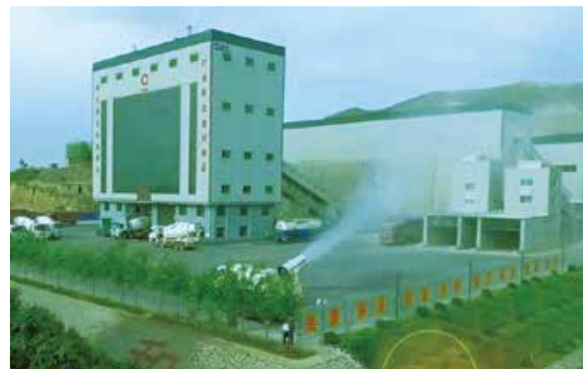
邢台中联2HLS180V (环保搅拌楼) 2HLS180V (environmental mixing tower) in China United Cement Xingtai Co.Ltd. (CUCC)
