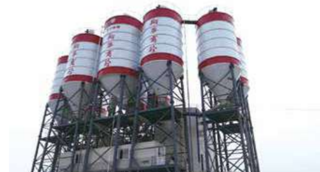
潮州翔华2HZS270V (商混站) 2HZS270V (concrete plant) in Chaozhou Xianghua
